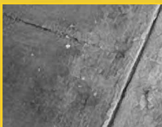
• Concrete Floor Joints
